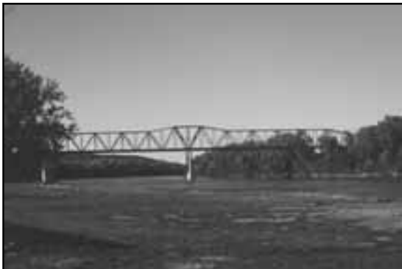
Bellevue Bridge over the Missouri River, SY02-116
