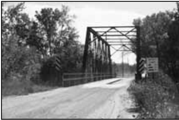
Pin-connected Pratt through truss near Gretna, SY00-193
