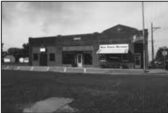
Mangold Building in Gretna, SY05-019
