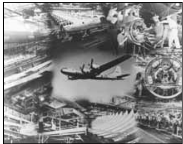
B-29 Superfortress production at Glenn L. Martin Plant, c.1944 (SCHS)
