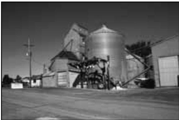
Grain elevator near Chalco, SY00-143
