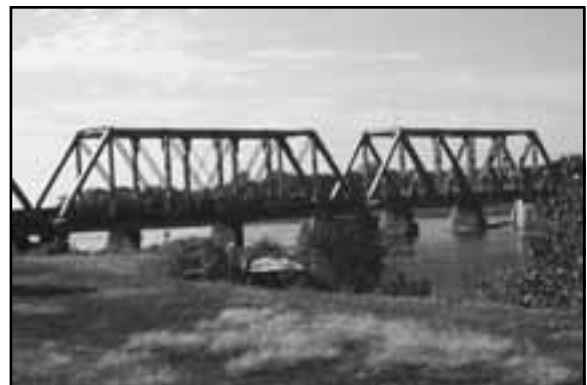
Railroad bridge near Bellevue, SY00-205
